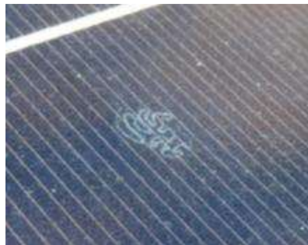
Glass antireflective coating delamination
